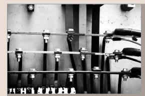
terminations in a completely enclosed, ventilated, protective metal housing. This assembly is designed to carry fault current and to withstand the magnetic forces of such current.
